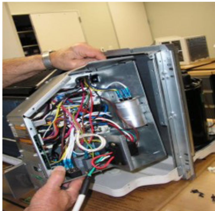
Figure 417 (Removal of Control Compartment)
