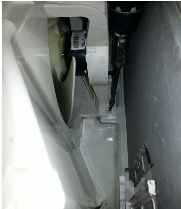
Figure 410 (Remove Gussets and Fan Shroud)
