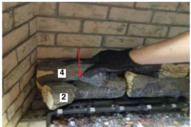
Diagram 10—Install Log 4
