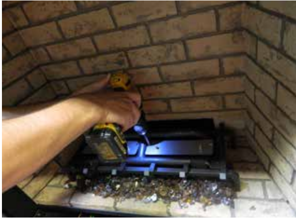
Diagram 5—Install Log support plates
