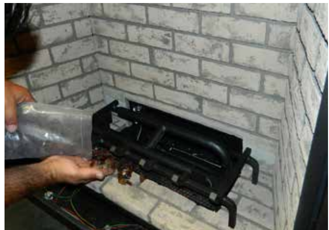
Diagram 3—Install Glass
