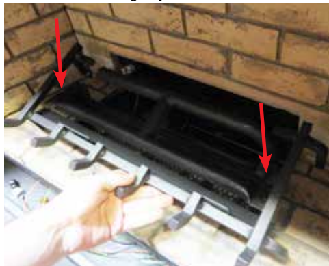
Diagram 1: Remove the left and right screws.
