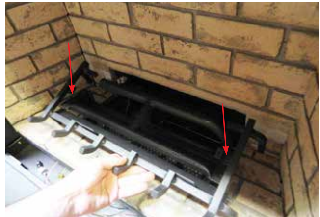
Diagram 2—Log Grate Install
