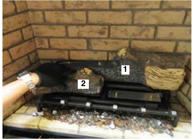
Diagram 8—Install Log 2
