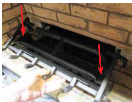
Diagram 1: Remove the left and right screws.
