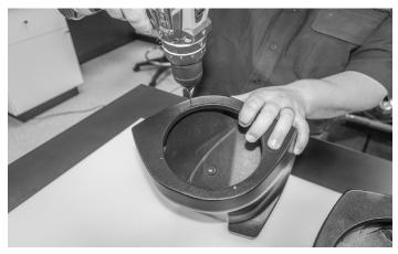
Next prep the speaker pods by drilling the holes in pods. The pods come with the mounting hole locations already marked. Use 1/8" bit to clean out the holes to prevent damaging the screws or enclosures.
