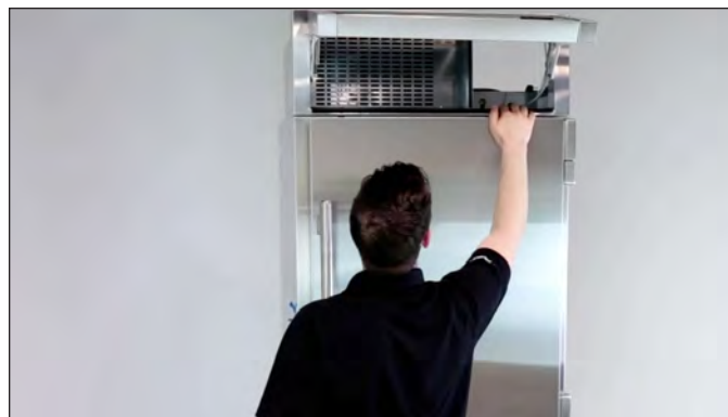
FIG. 3. Be sure to inspect behind the rainshield.
