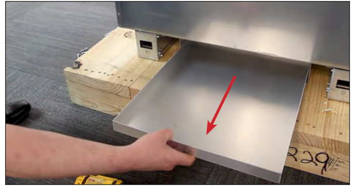
FIG. 9. Remove the drain pan before pulling the appliance off the skid.
