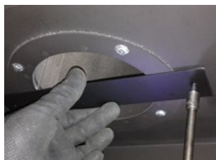
Figure 8.b.c Restrictor plate Installation
