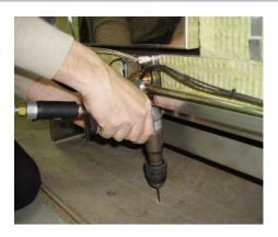
4. Where the floor consists of tiles, concrete or another hard material, drill a 10 mm diameter hole, push in the plug and screw the stud into it.
