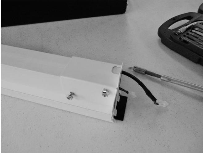
Attach the right hand mounting bracket to the new mullion assembly.
