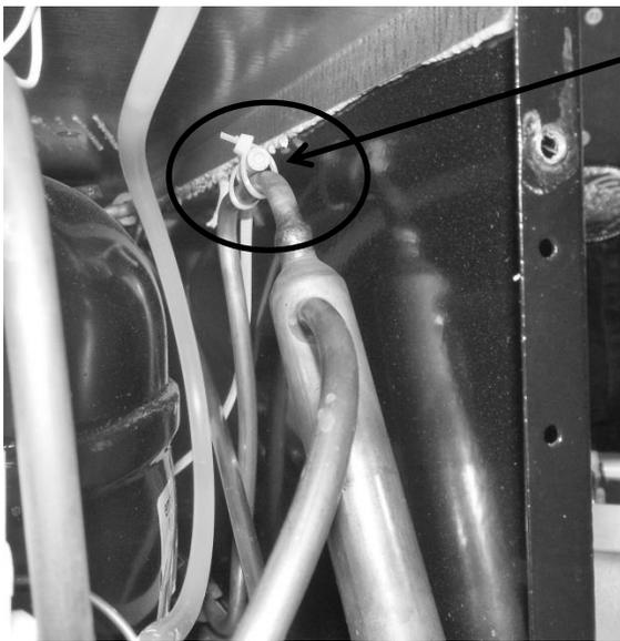
High side thermistor location: The thermistor is fastened to the liquid line at the filter drier with a nylon wire tie.
