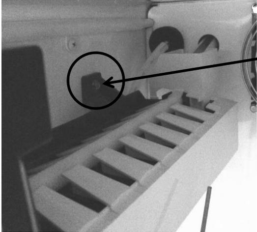
Set the Ice maker on top of each of the (two) top screws and tighten.
