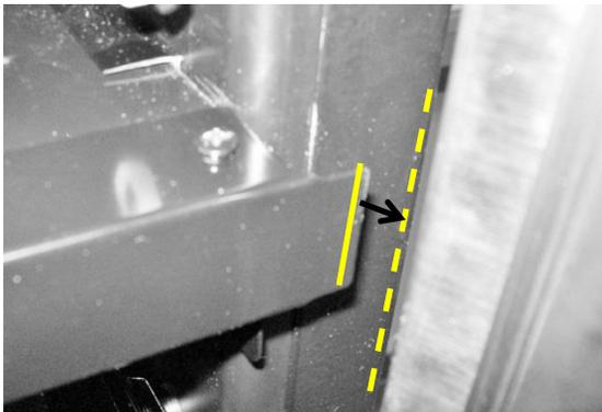
Once the mullion face is removed, the divider can be slid forward and out of the cabinet.
