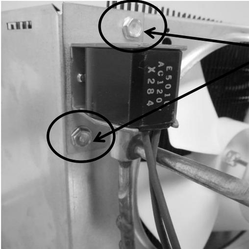
The hot gas valve is secured with two 5/16" sheet metal screws.
