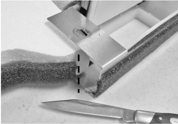
Cut the foam insulation on each side of damper bracket.
