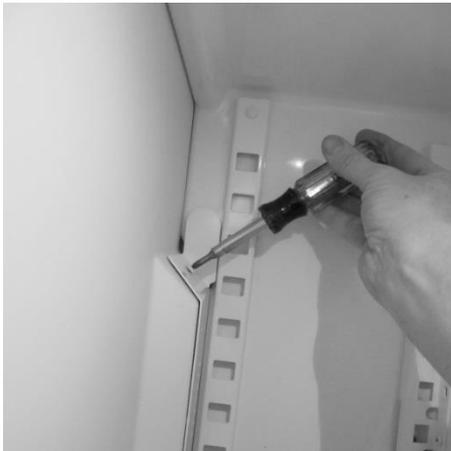
To access the damper, remove all three screws from the cover face.
