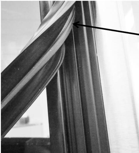
Press the gasket foot into the door channel to reseal. Use your thumb to work the gasket in place around the perimeter of the door.
