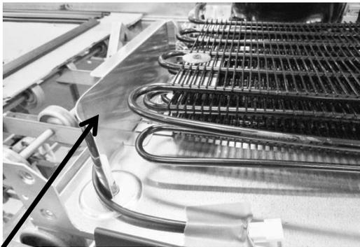
**NOTE:** On machine compartments with LEFT HAND SWING doors, a shield is added to prevent the communication cable from being drawn into the condenser coil. It is anchored using the same nut which secures the condenser mounting bracket.
