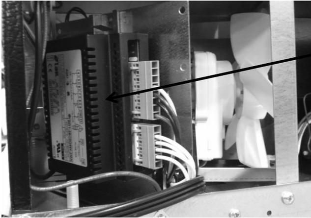
**Main Power Board** – Located in the left hand side of machine compartment.
