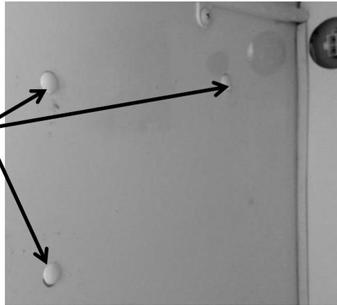
Install screws into the top two holes; leave room to set the ice maker into place on top of screws.
