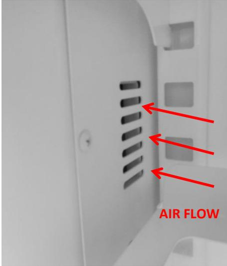
Air transfer damper is located behind this louver cover.
