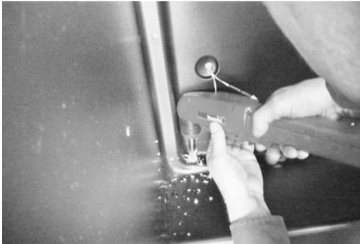
**Drill a ½" hole downward into machine compartment.**
