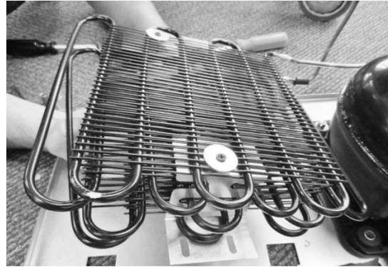
Condenser can be lifted away from bottom assembly after following step 7 above.
