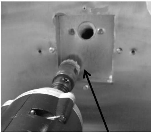
Use a 1" hole saw to completely drill through the bottom left hand corner inside the water fill tube recess.
