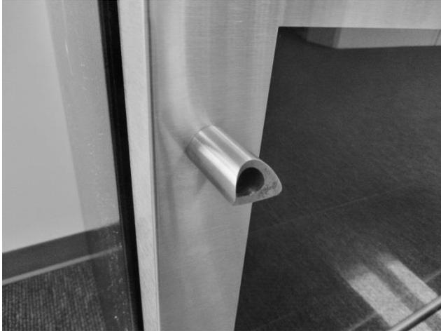
If the standoff is loose it can be tightened with a Phillips screwdriver.
