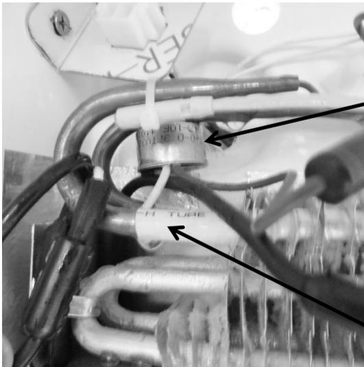
The Termination thermostat is located on the evaporator outlet.
