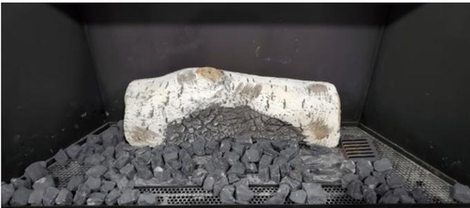
**Step 2:** Log **G** is placed in front of the pilot at the right end of log **A**
