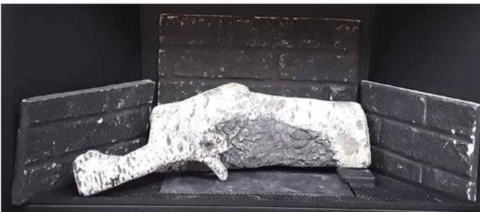
**Step 3:** Log **F** is placed resting on log **A** and behind log **E**
