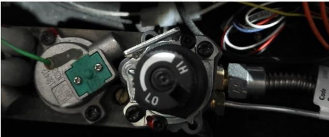
**Figure 13.ee** LP pressure regulator on a Basic
