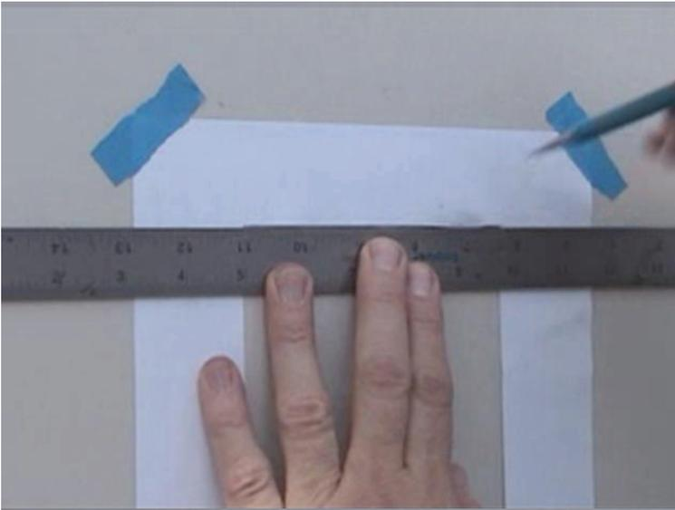
Mark the wall with the required cutout dimensions for the James model you are installing. Keep the vertical lines plumb so the speaker will be straight when installed. A level should be used.
