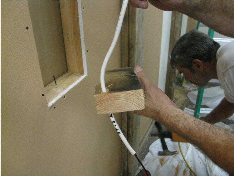
Also, if you are fully boxing in the wall opening, you might want to drill a hole in the top 2x4 and fish your wire through so the final 2x4 can be placed.
