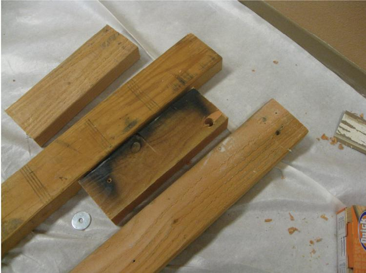
The wall board will not support a large BE series directly without additional support. So the cutout should be boxed in with 2x4 to provide something for the mounting screws to fasten to.
