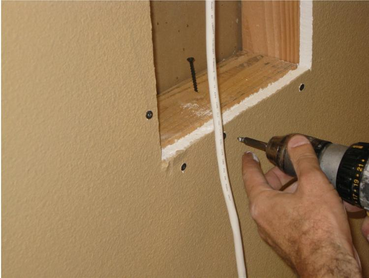
While holding the drywall screw “handle”, screw through the drywall into the 2x4’s with dry wall screws. Be sure NOT to place screws where you previously marked the speaker mounting holes or you will not be able to mount the speaker later.
