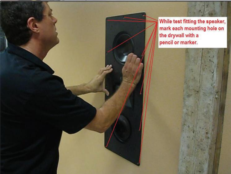
While test fitting the speaker, mark each mounting hole on the drywall with a pencil or marker.
