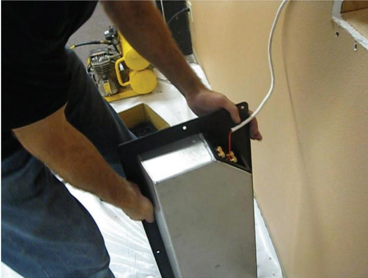
Connect the speaker wire to the speaker terminals observing polarity markings.
