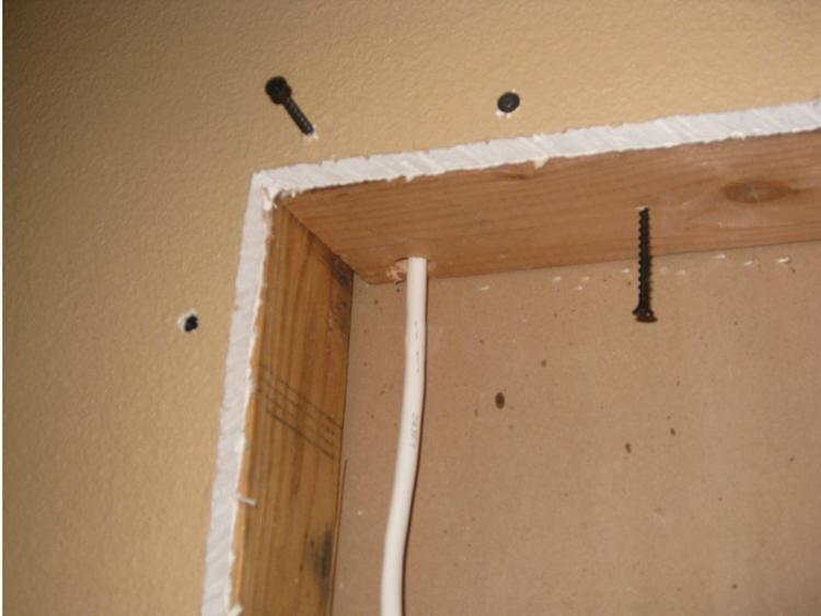
Shown here is the top 2x4 with the speaker wire fished out and the last drywall screw being placed to hold the 2x4. The “handle” screw is still in the top 2x4 and will be removed.
