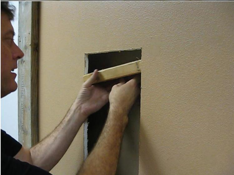
While holding the drywall screw "handle", slide the 2x4s into each location.
