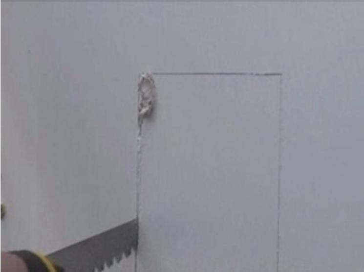
After Marking the wall, use your preferred method of cutting the hole, either using a power tool or by hand.
