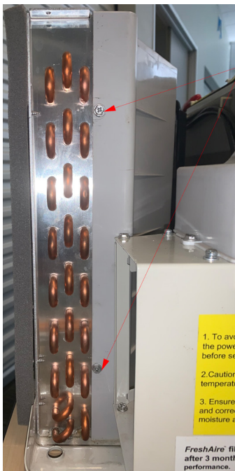
Figure 532 (Remove Brackets and Shroud)
