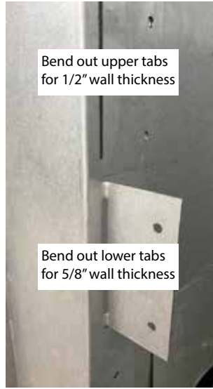
Figure 6.4 Nailing tab bent out for installation
