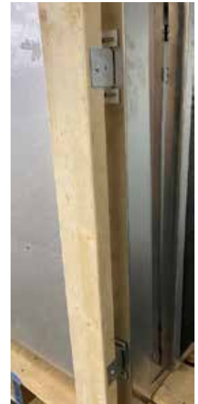
Figure 6.8 Fasten installation brackets to wall framing
