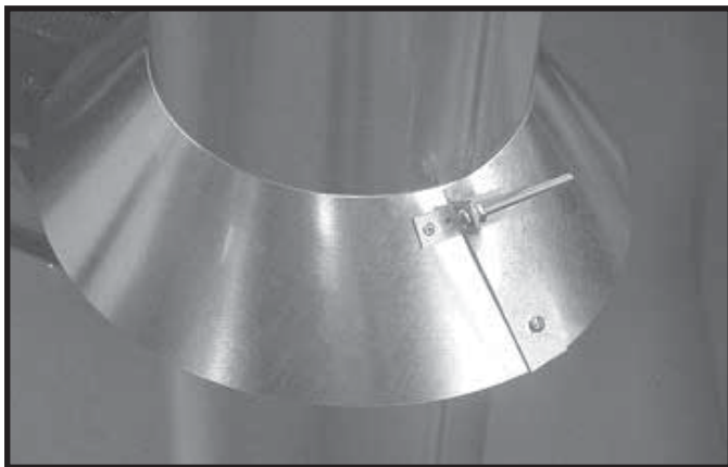
Figure 7.13 insert Bolt into Brackets
