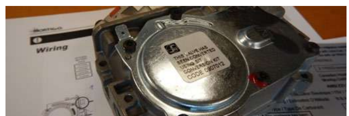
Figure 13.k Conversion label on valve
