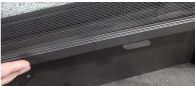
Figure 20.b Lift out the Retaining Tabs and screen
