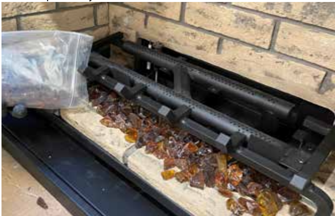
Diagram 3-Install Glass
