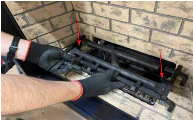
Diagram 2-Log Grate Install
