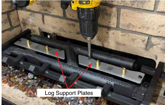
Diagram 5-Install Log support plate installation
