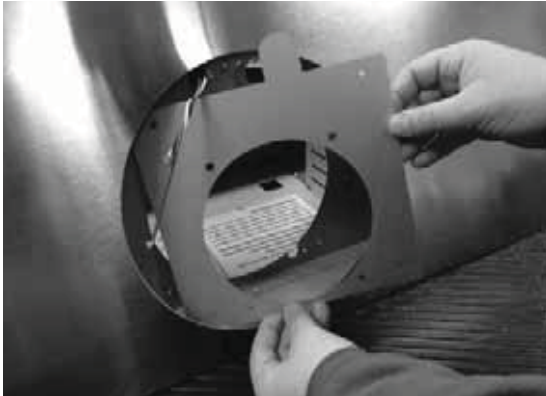
1. Remove internal blower flange plate.
