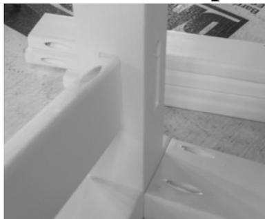
Align back slats in between legs with pocket facing up. Tap into notches on each side of the leg. Secure using (2) 1-1/4" Phillip's head screw. Attach one back slat at a time from the bottom up. Repeat process for all back slats.
