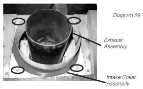
12. From the outside rear of the firebox: install the intake cover plate with 4 - 1/4" x 1/2" screws. Ensure all screws are tight, but do not over tighten. All 4 screws must be used.
