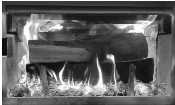
Close the primary air control by small increments (ex: 1/16 of an inch) until reaching 1/4in before closed position, between 4 and 15 minutes after the loading period. Before closing further, make sure the flame intensity is increasing or stable. Turn ON the blower at minimum speed after 30 minutes.
