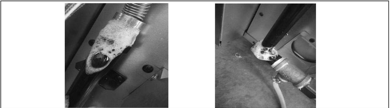
**⚠WARNING** DO NOT use a flame to check for gas leakage.
