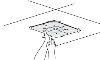
3. Use a pencil to mark the mounting screws, wire access and duct hole locations on the ceiling.
