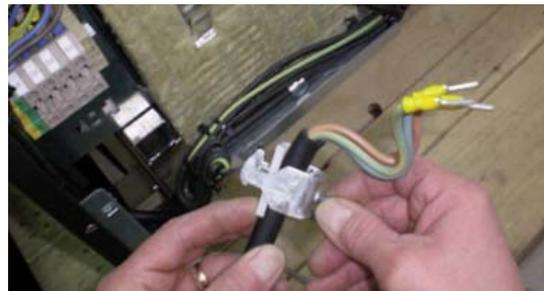
4. Insert the strain relief device into the hole and push it to the left. Tight up the power cord and strain relief device with the screw.
