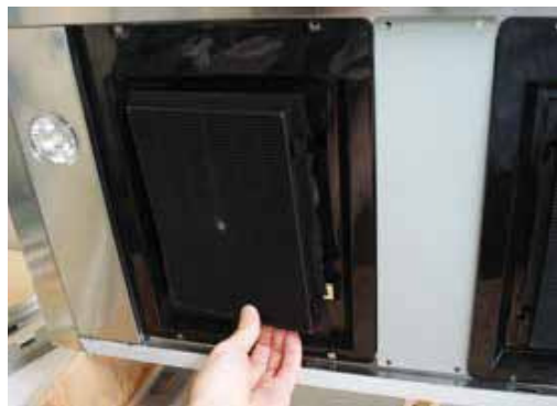
3. Install charcoal filters into charcoal filter brackets
