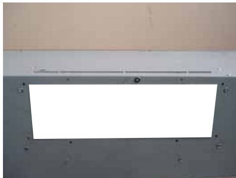
Horizontal Ducting (3-1/4"x10" Rectangular)
