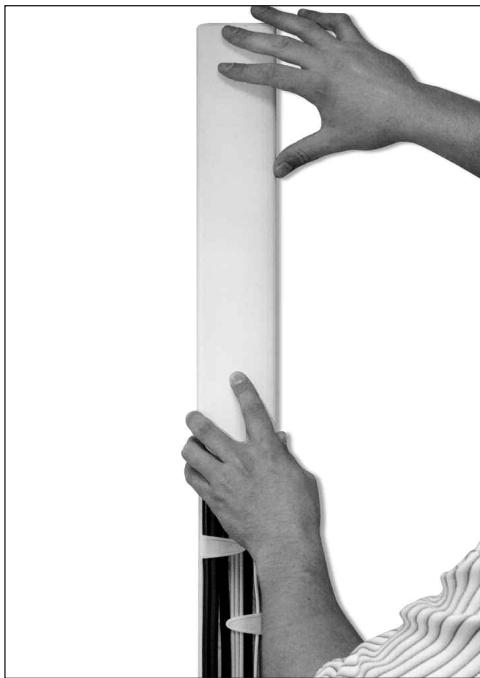
4-1. Starting at the top, snap on the first wall track cover (AA). Make sure the top of the cover aligns with the top of the wall track (A).
