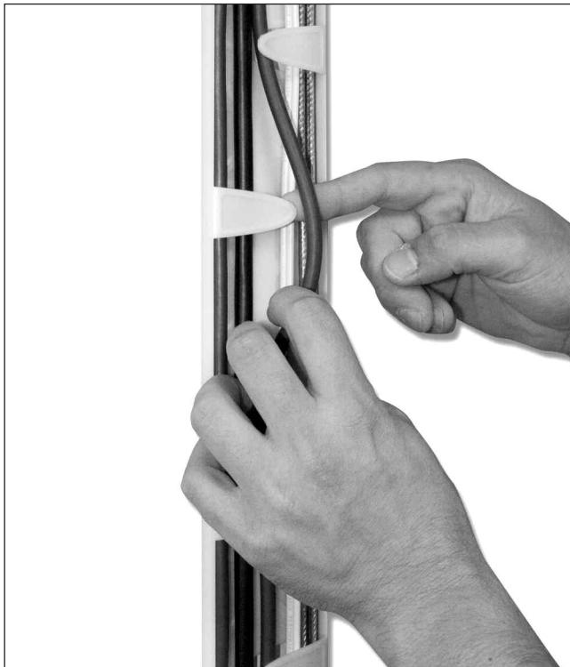
3-1. Check your installation to make sure there is nothing that could cut or damage your cables. Starting at the top, route the cables through the wall tracks. Be careful not to kink the cables.
