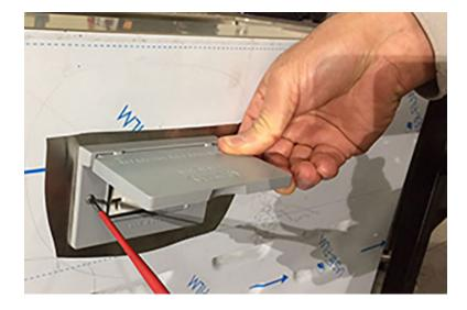
Install the foam gasket, and weather-proof cover with the screws provided.
